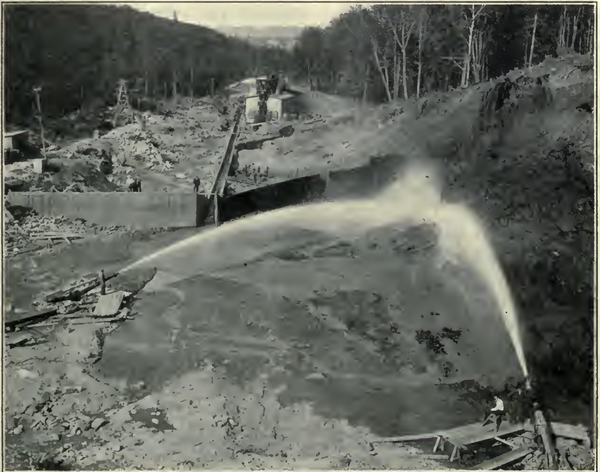
HYDRAULICKING AT BEAUCEVILLE, QUEBEC.
